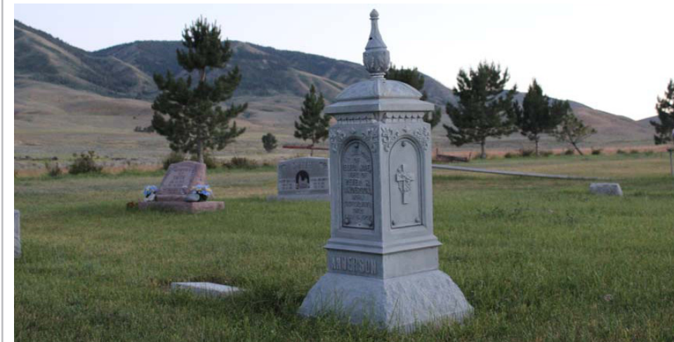
Above is a pre-fabricated zinc monument found in the Samaria, Idaho cemetery. These zinc markers were manufactured in Bridgeport, Connecticut from the 1870's through 1912 (Photo: Lisa Duskin-Goede).
